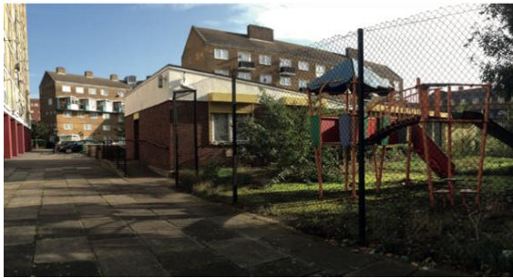
View of derelict nursery building (Images: Bell Phillips Architects)
